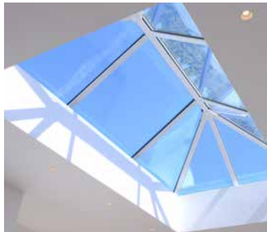
STEEPER ANGLE FOR SMALLER ROOFS
